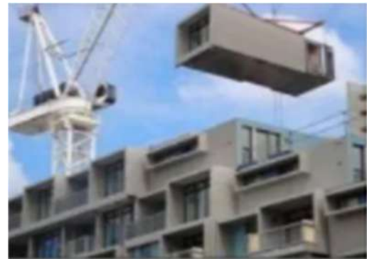
Fig 86: Volumetric Construction
