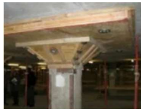
Fig 87: Flat Slab Construction
